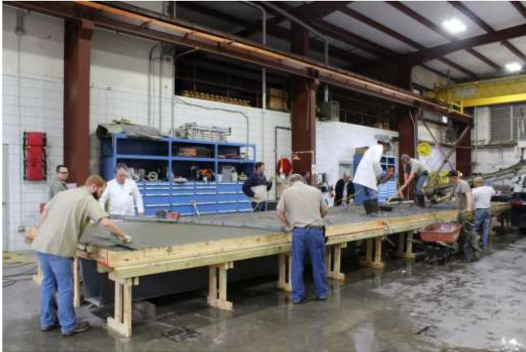
**Figure 3-9 Casting the concrete deck.**
