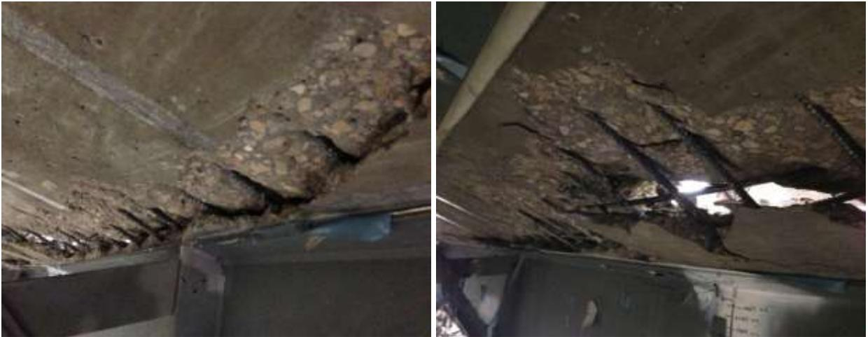
**Figure 4-20 Punching in the bottom of the deck.**
