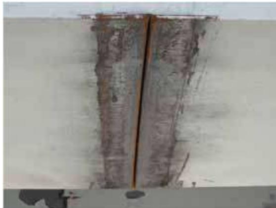
**Figure 1-3 Bottom flange cut after the explosion (Source: FHWA Report No FHWA/TX-10/9-5498-1).**
