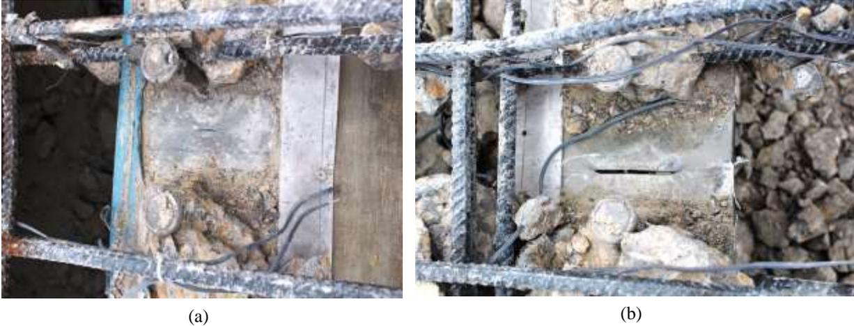
**Figure 4-33 Damage in (a) the inner top flange, (b) the outer top flange of the damaged girder.**
